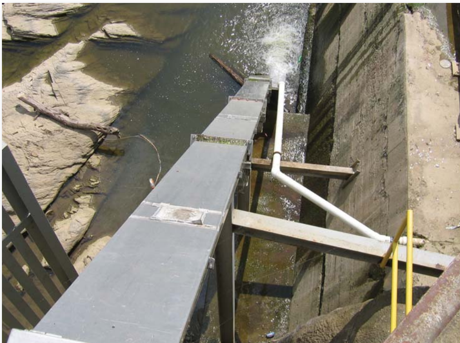
Eel ladder on Shenandoah River. The round, white pipe releases water from upstream, attracting eels to the ladder. The metal ladder has fabric inside which the eels crawl up.
